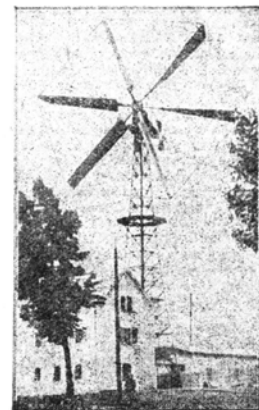
A typical installation that provides a 2000 acr farm with electricity.
