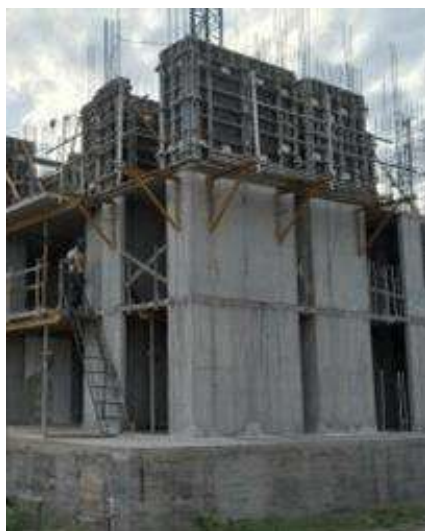
Figure 1. Typical concrete structure
