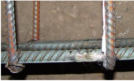
Figure 3. Surface cleaning, installation of strainsensors and epoxy resin protection
