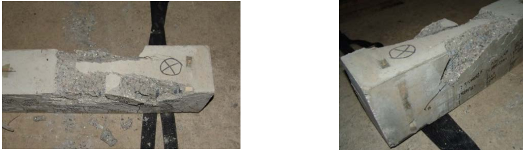
Figure 8. Representative beam destruction
