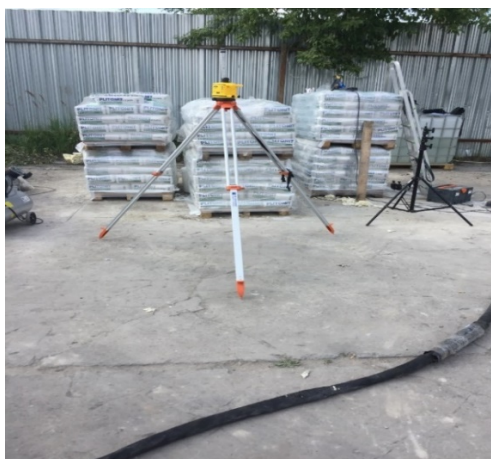
Figure 5. The injected plot under the load during the injection process
