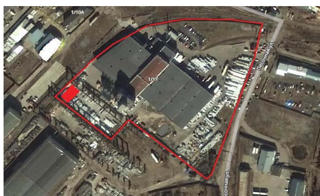
Figure 1. The layout of the object (the red Line highlighted the boundary of the plant; red fill indicates the test area)
