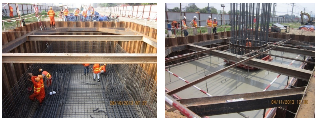
Figure 1. Construction of the foundation's bridge in Vietnam
