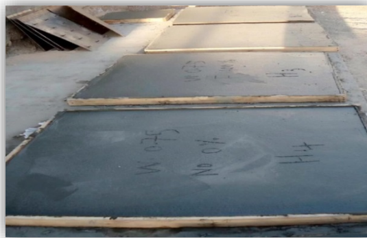
Figure 3. Slabs after casting.
