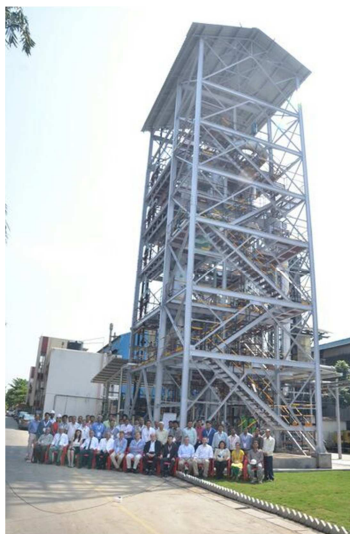
Fig. 4. 1 MW circulating fluidized bed gasification facility developed within the EU OPTIMASH project.
