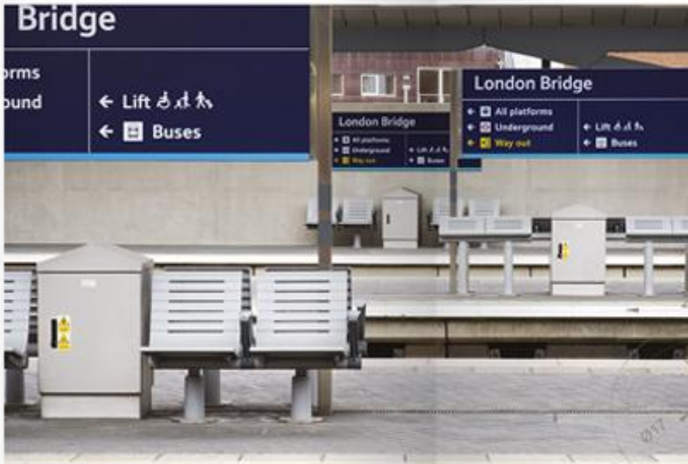
The benches are equipped with a wheelchair access point.
