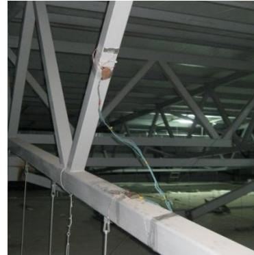
Figure 6. Installation of strain gauges on the truss rods
