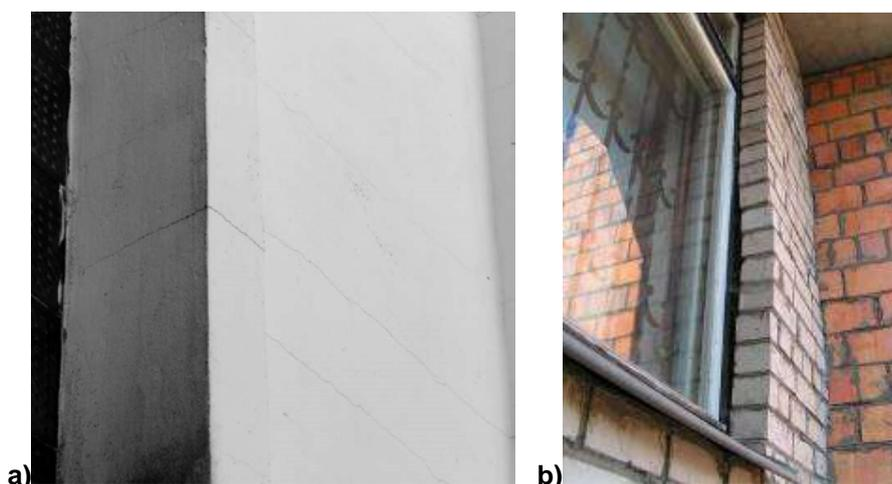
**Figure 1 - Typical damages of eccentric-compressed masonry walls:**
