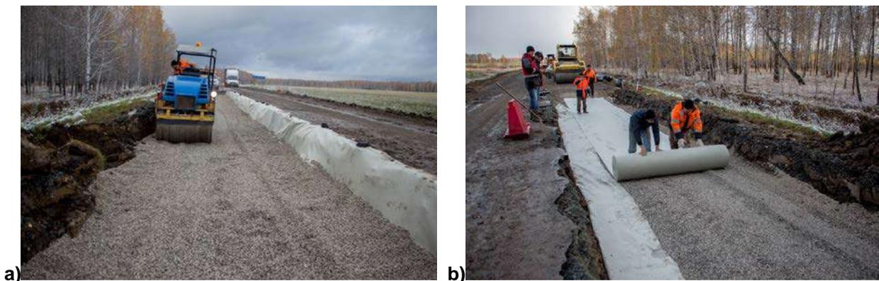
Figure 6. Construction of the experimental section with GC: a – GC compaction by roller; b – geotextile laying above GC
