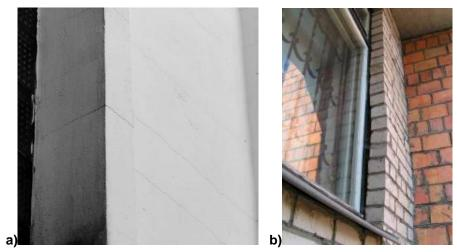
Figure 1 - Typical damages of eccentric-compressed masonry walls: a) horizontal cracks on the tensile surface of the partition wall; b) loss of stability of the facing layer of masonry
