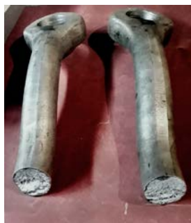
Figure 1. Fatigue fracture of the element of the load-lifting device of the construction crane
