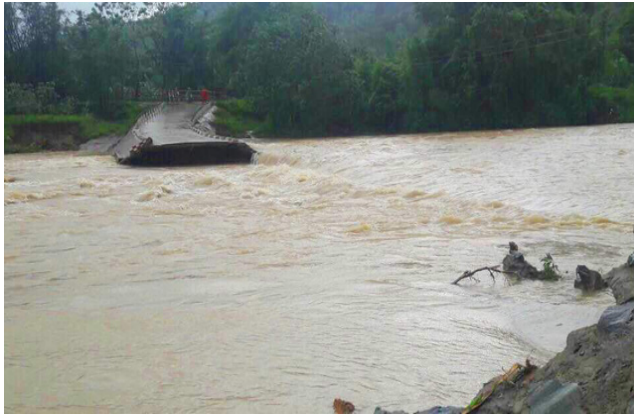
Figure 1. A-Sap bridge collapsed in Thua Thien Hue province, Vietnam, November 2016.
