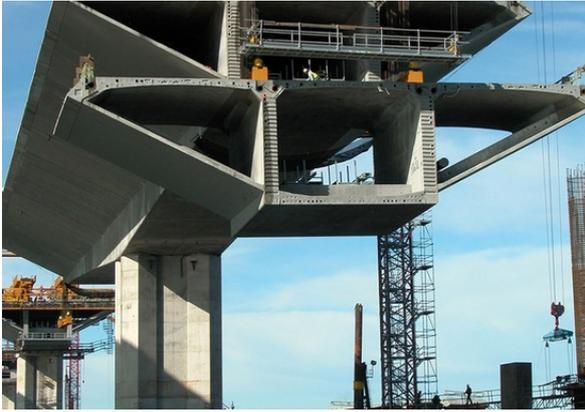
**Figure 1. Box-girder bridge multi-cell cross-section [23].**
