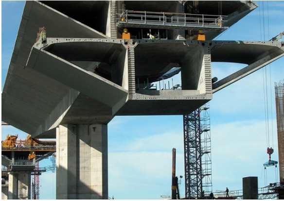
Figure 1. Box-girder bridge multi-cell cross-section [23].
