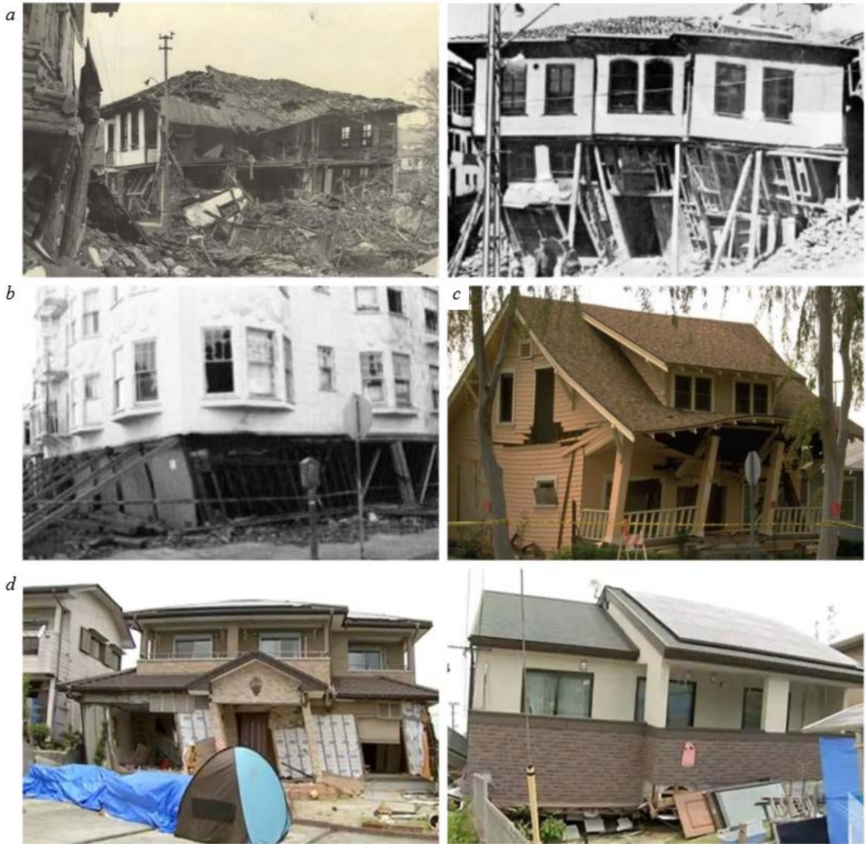
Figure 3. Examples of timber frame building failures: a – March 1970 Geiz (Turkey) [8–9]; b – earthquake in San Francisco (USA) in 1989; c – earthquake in Norwich, California (USA), in 1994 [10]; d – earthquake in Kumamoto (Japan) in April, 2016 [7].
