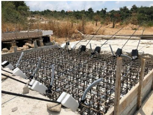
Figure 10. PT-1R slab before the concrete cast.
