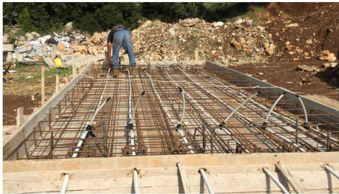
Figure 2. PT slab execution.
