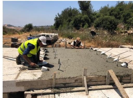
Figure 11. Concrete cast for PT-1R.
