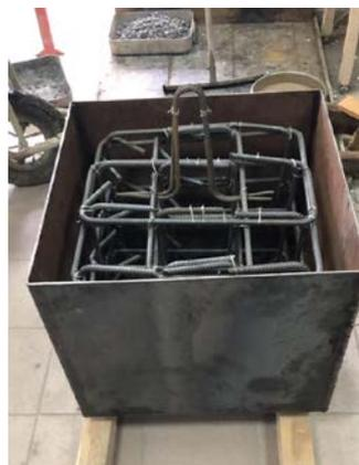
Figure 4. RC block reinforcement (cm).
