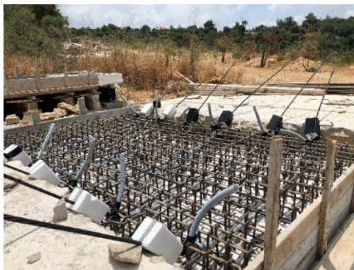
Figure 10. PT-1R slab before the concrete cast.
