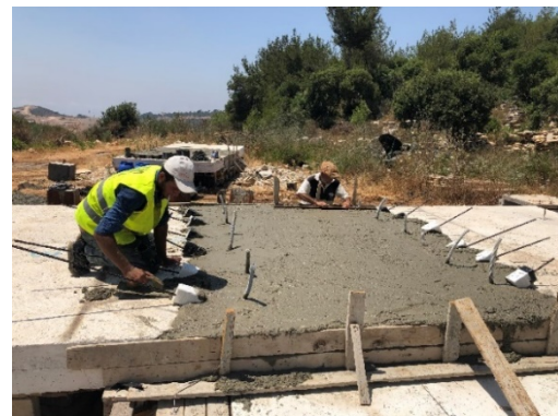
Figure 11. Concrete cast for PT-1R.
