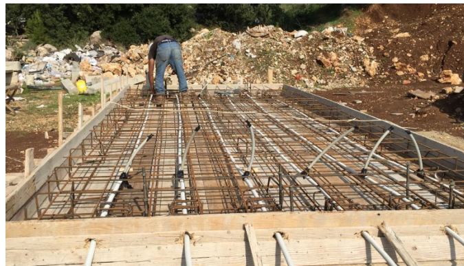
Figure 2. PT slab execution.
