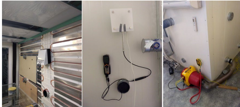
Figure 1. The experimental setup – air intake from the simulated cold outside conditions through integrated wind protection frame (on the left); air supply side in the warm room (in the middle); ventilator, which generates the simulated overpressure in the climatic chamber (on the right).
