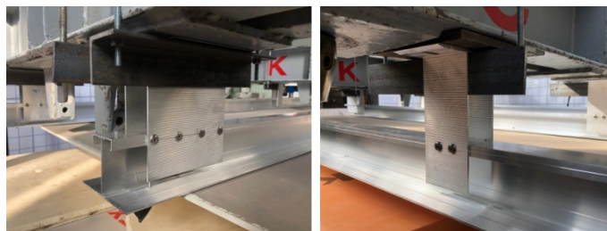
Figure 4. Attachment of brackets to traverses and fixation of the subframe to the brackets.
