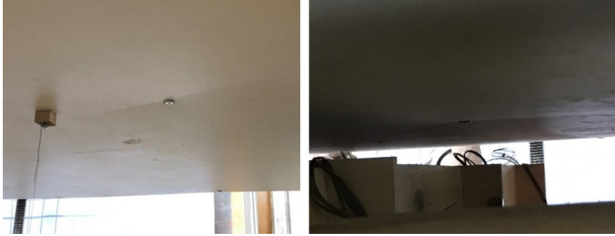
Figure 15. Crack formation: left – sample 1 under the load of 155.56 kg/m 2 ; right – sample 2 under the load of 200 kg/m 2 .
