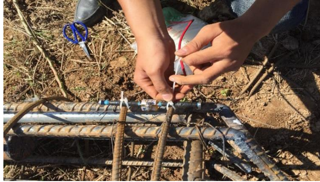
Figure 4. Strain gage for measuring concrete displacement.
