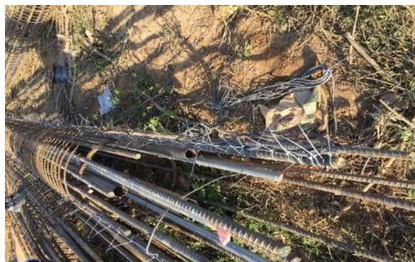
Figure 3. Extensometer equipment for measuring the displacement of pile.
