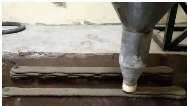
Figure 6. 3D concrete printing process.
