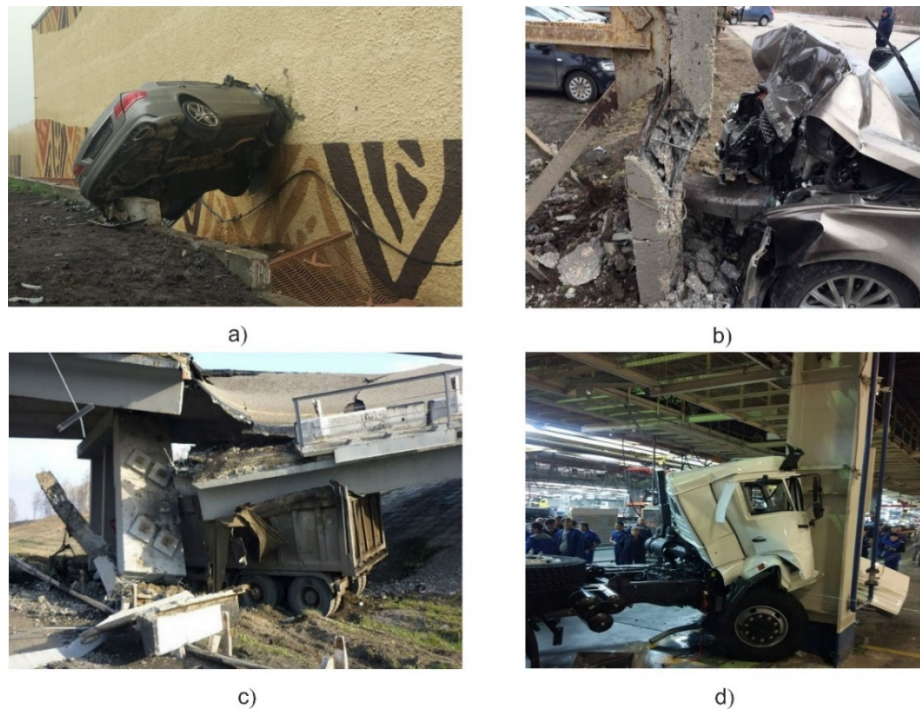
Figure 1. Emergency actions on structures: a) impact with preservation of static force after action; b) local damage with partial exclusion of the pillar from work; c) the complete exclusion of the column, followed by the interaction of the structure with the deformable barrier; d) local damage without removing of the element.
