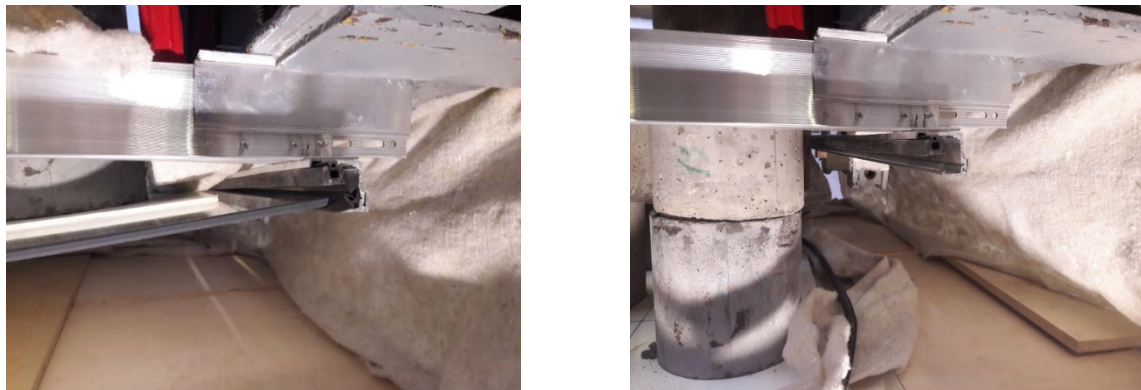
Figure 29. Deformation of sealant (test setup 1).
