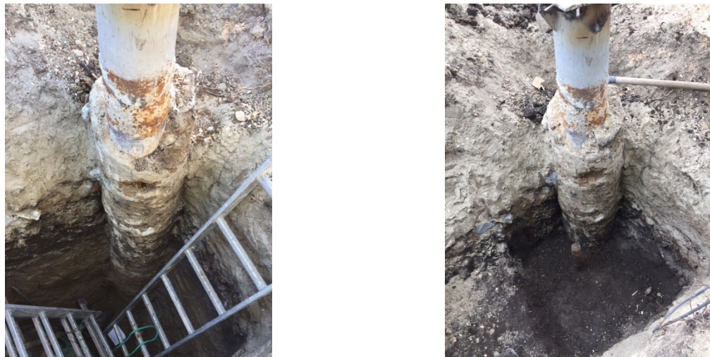
Figure 9. A “soil shell” along the pile perimeter.
