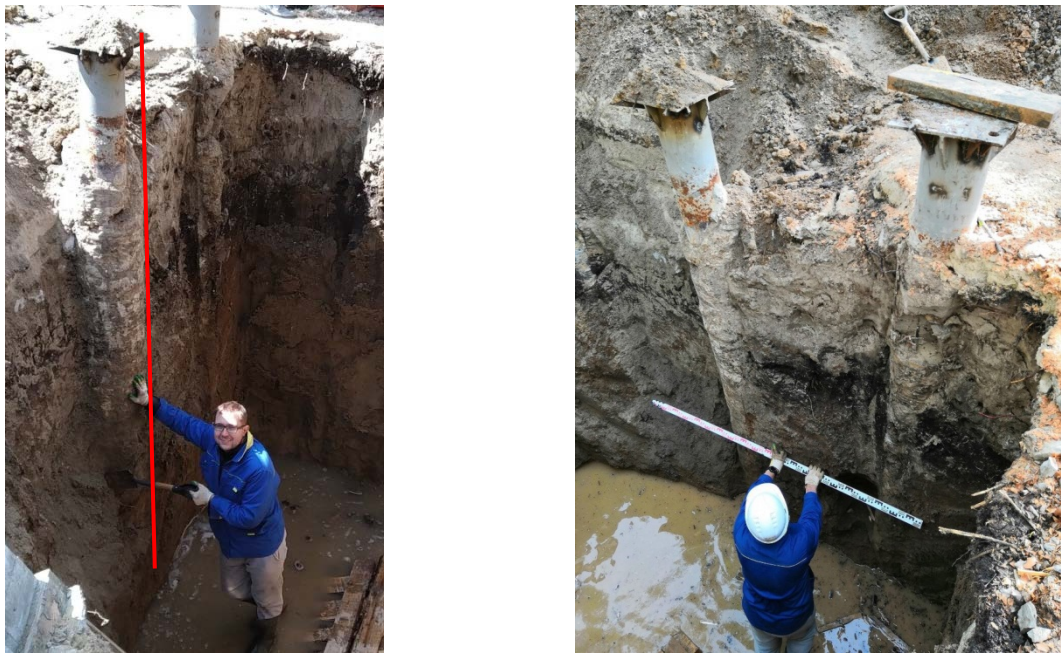
Figure 8. Drill-injection piles inspecting.
