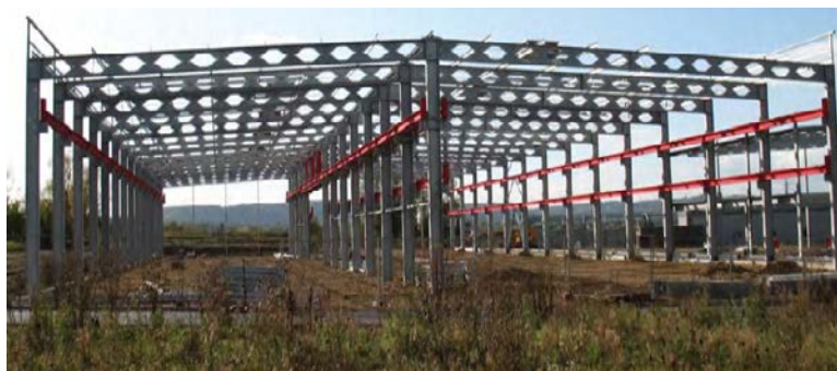
Figure 1. Framework with sinusoidal perforated beams.
