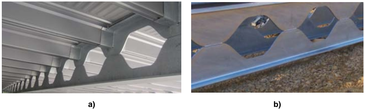
Figure 6. Perforated beams with different fillet radius of corner: a) r = 0.25a ; b) r = 0.75a .
