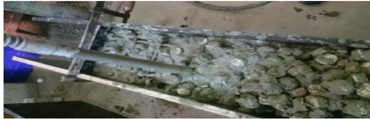
Figure 6. Casting and compaction.
