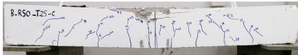
c) B-R50-T25-C, Loading cracks
