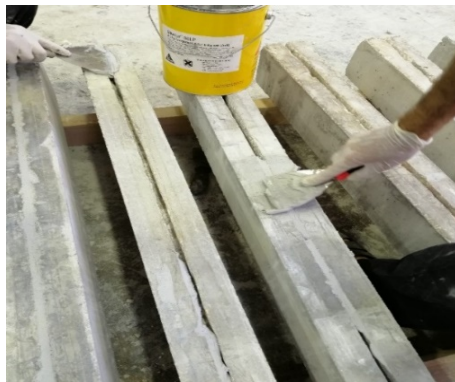
(c) Filling the grooves with "epoxy" paste
