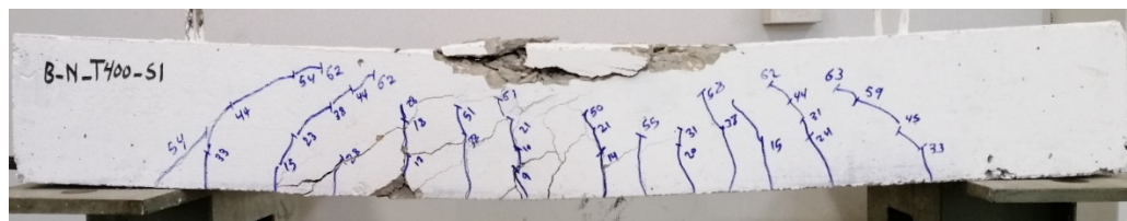
a) B-N-T400-S1, Loading cracks
