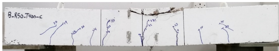
c) B-R50-T400-C, Loading cracks
