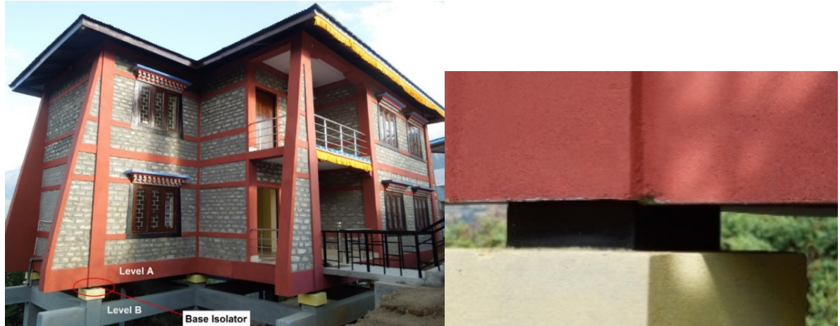
Figure 1. A view of the prototype base-isolated building [17].
