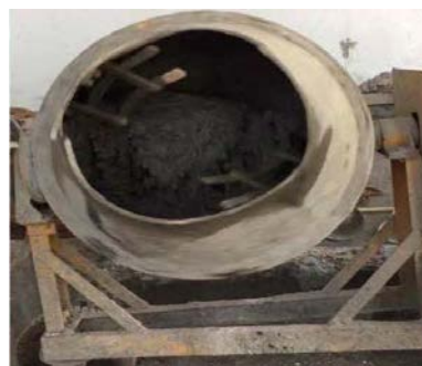
Mixing concrete by tilting drum mixer
