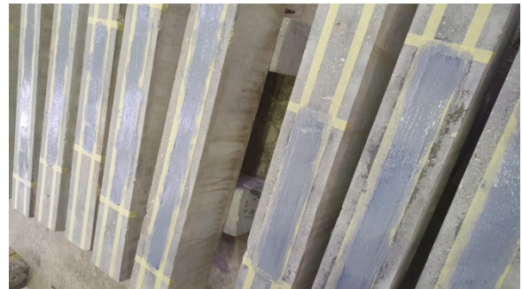
Applying the two layers of epoxy onto CFRP sheets surface
