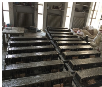
Casting concrete into molds
