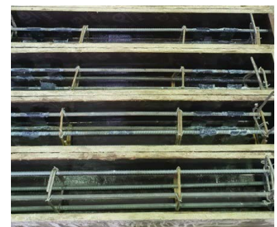
Wooden mold for casting beams
