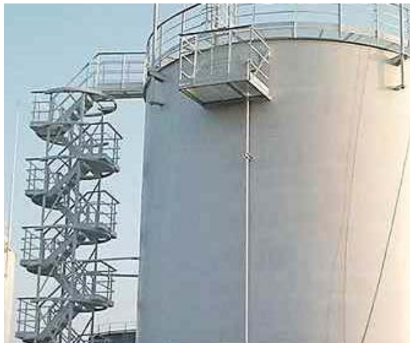
Figure 1a. Tank stair tower.
