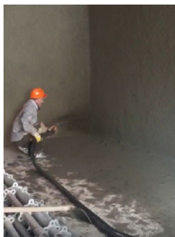
Figure 9. Strengthening a structure with shotcrete.
