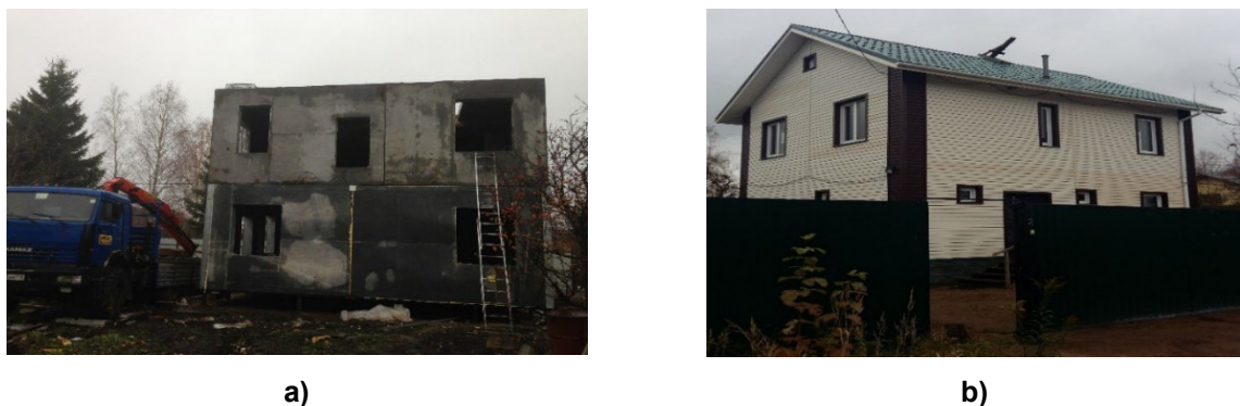
Figure 2. a) Mounted panels of a LSCS house on the 5 th day of construction; b) Finished house on the 15 th day of construction.
