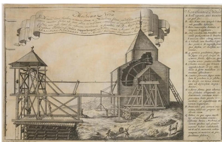
Figure 1. Christopher Polhem's hauling engine or hoist, the Machina Nova, at the Falu copper mine, Sweden. This hydro-powered construction dates to 1694 (cc BY-NC-ND Nordiska museet/Sverige Dalarna Falun, Photo Peter Segemark – url digitaltmuseum.se )
