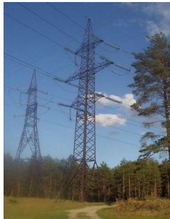
Figure 1. General view of the anchor-corner support of a 220 kV OHPL.
