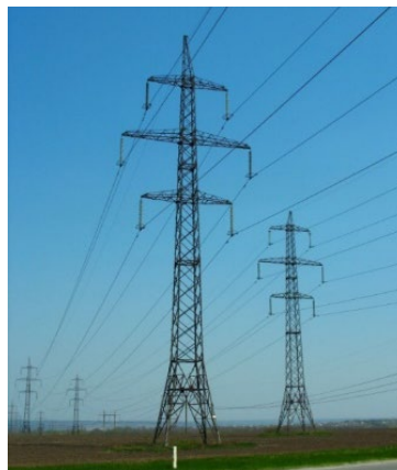
Figure 2. General view of the intermediate support of a 220 kV OHPL.
